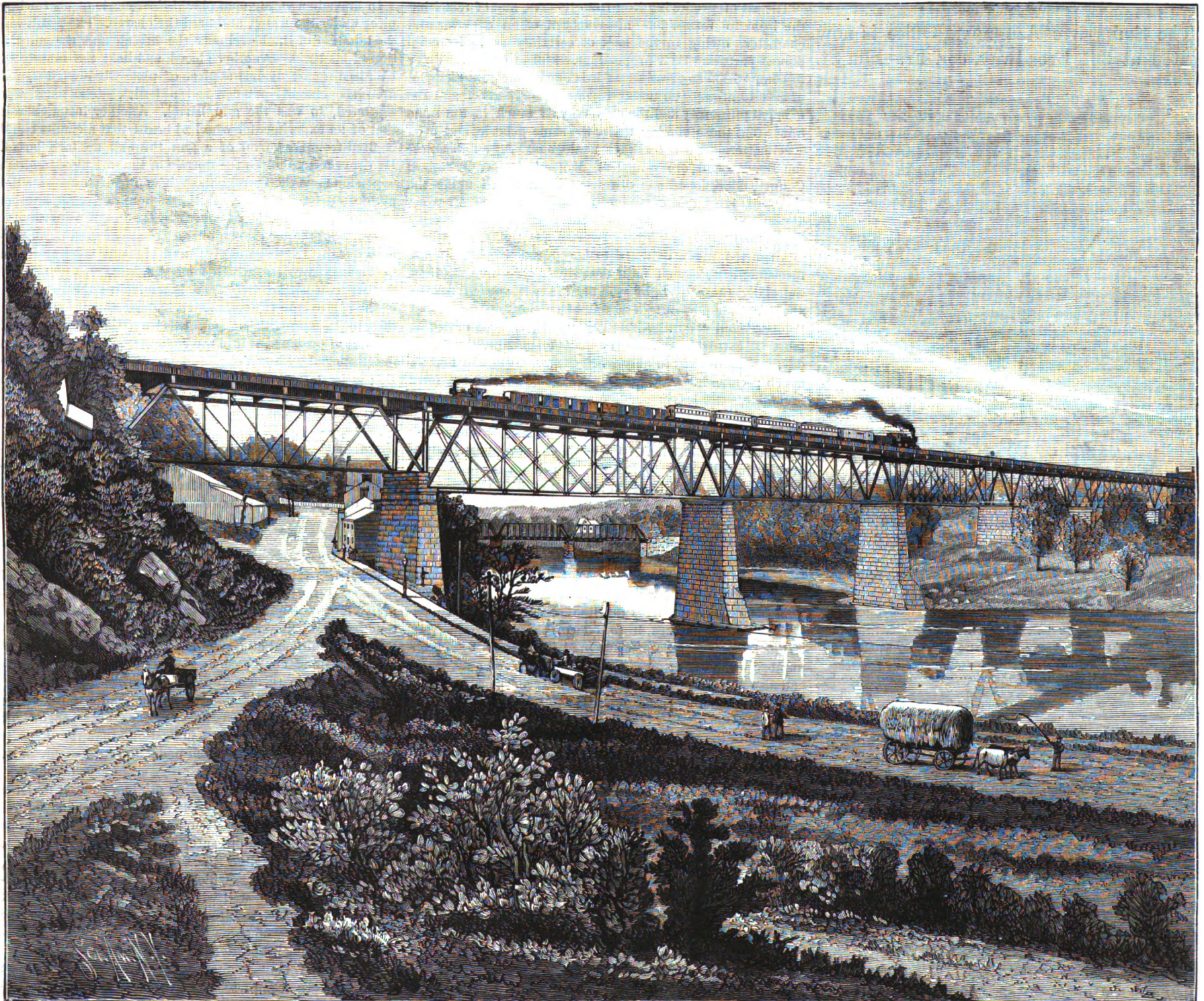
VIEW OF CATSKILL CREEK BRIDGE, ON THE N. Y., W. S. & B. R.R., LOOKING TOWARD THE HUDSON.
