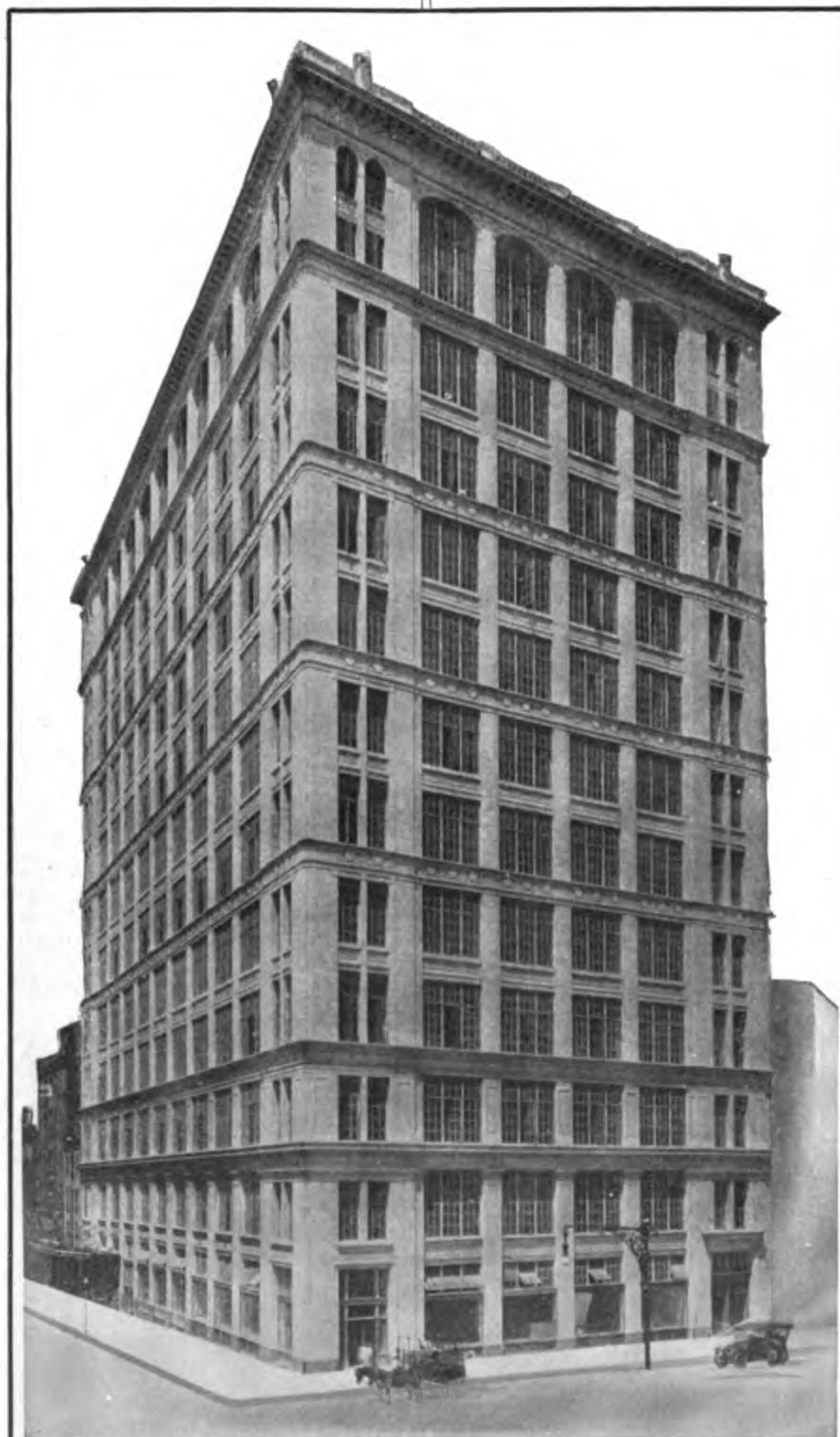
THE HILL BUILDING New York's Most Modern Publishing Building, at Tenth Avenue and Thirty-sixth Street, New York
