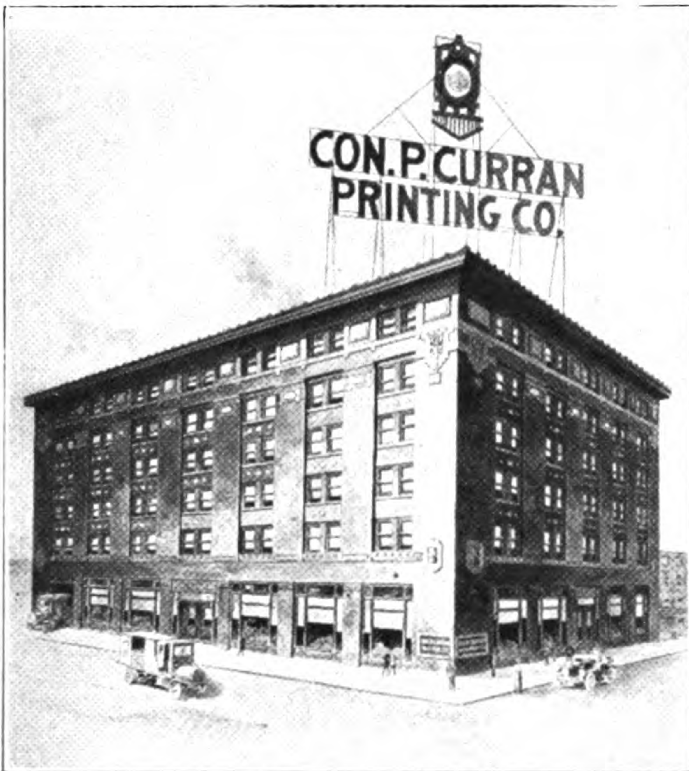
Curran Building, at Eighth and Walnut Sts., St. Louis, Mo.
